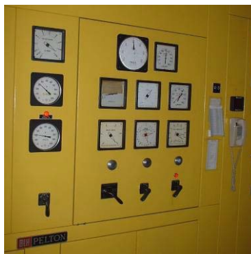
Figure 5: A legacy governor conversion candidate at the USACE Little Goose plant (Washington) – Pelton mechanical cabinet actuator
