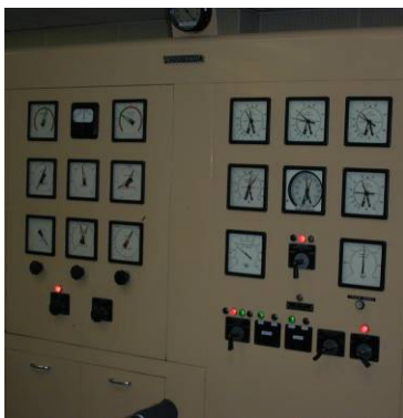
Figure 4: A legacy governor conversion candidate at the USACE Detroit plant (Oregon) - Woodward mechanical cabinet actuator
