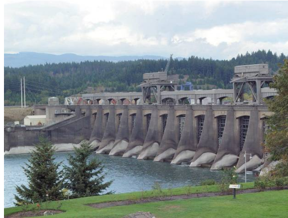
Figure 3: USACE Ice Harbor hydroelectric plant in Washington
