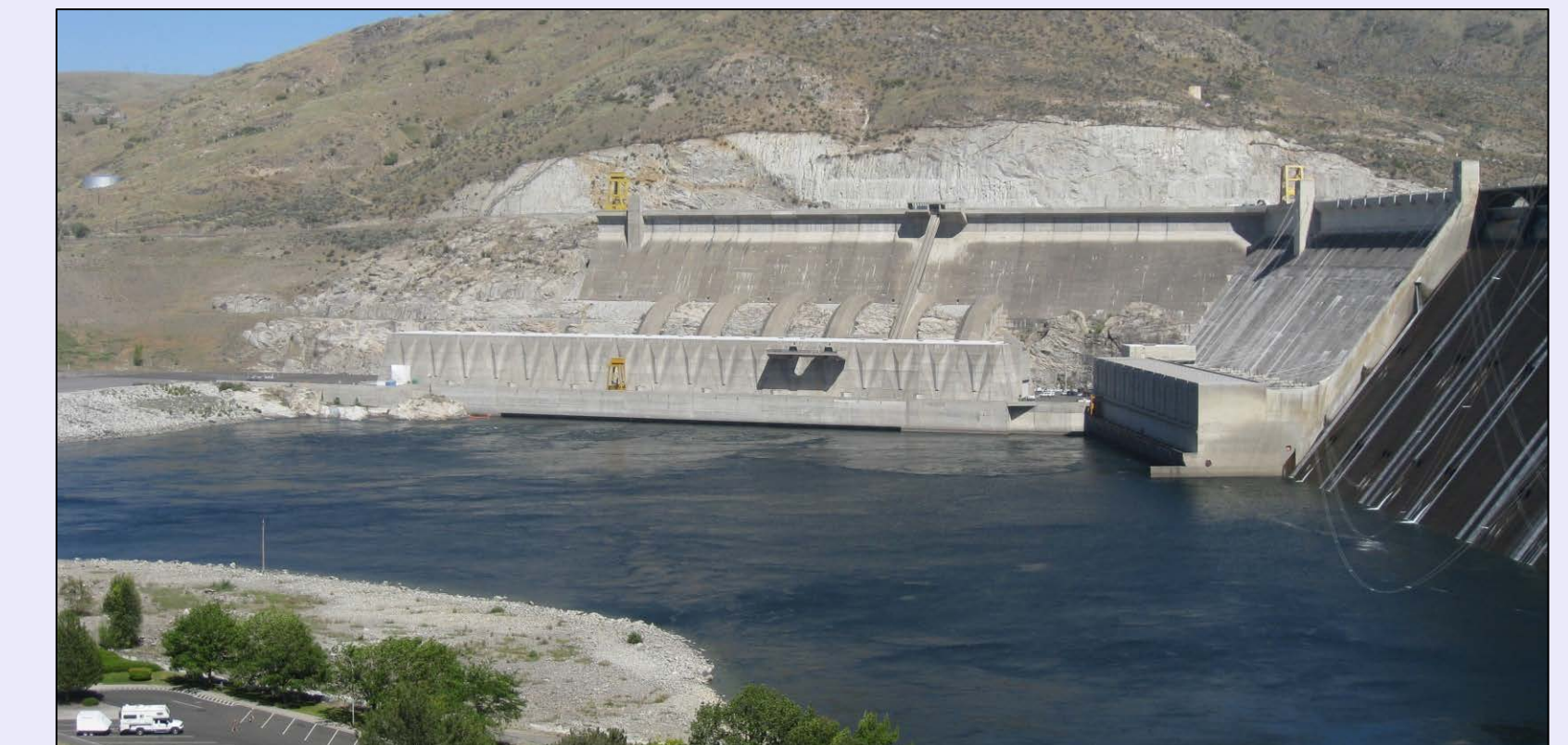
Figure 10. The Grand Coulee Third Power Plant (Center). The Right Power plant and the main dam spillway are shown on the right.
