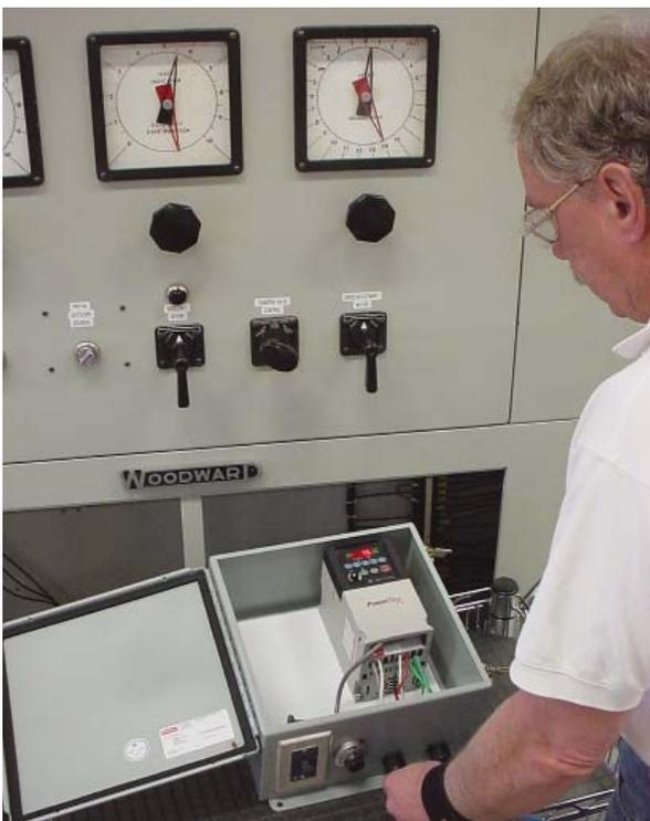
Pacific Gas and Electric Company personnel use ballhead drive simulators to perform on-line calibration of mechanical governors when other work being done on the turbine or generator prevents the unit from operating.
