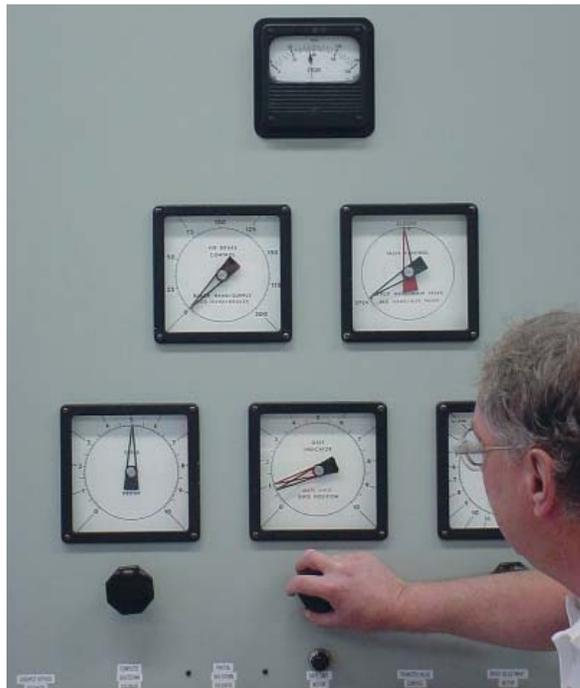
During on-line calibration of the mechanical governors, Pacific Gas and Electric Company personnel test stability by introducing a speed/frequency disturbance using the gate limit and watching how the governor responds.
