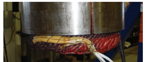
PMG Stator Lead Repair – After
