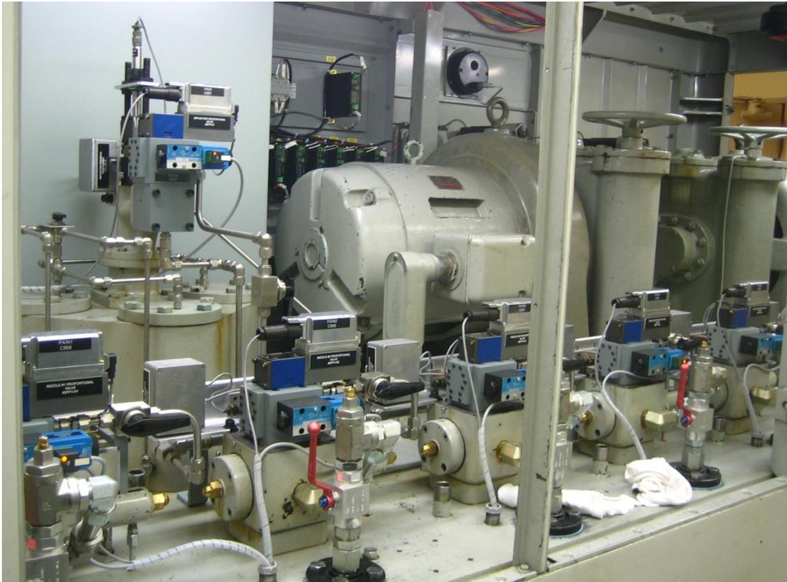
Figure 7 – New Deflector and (6) Needle Hydraulic Control Manifolds
