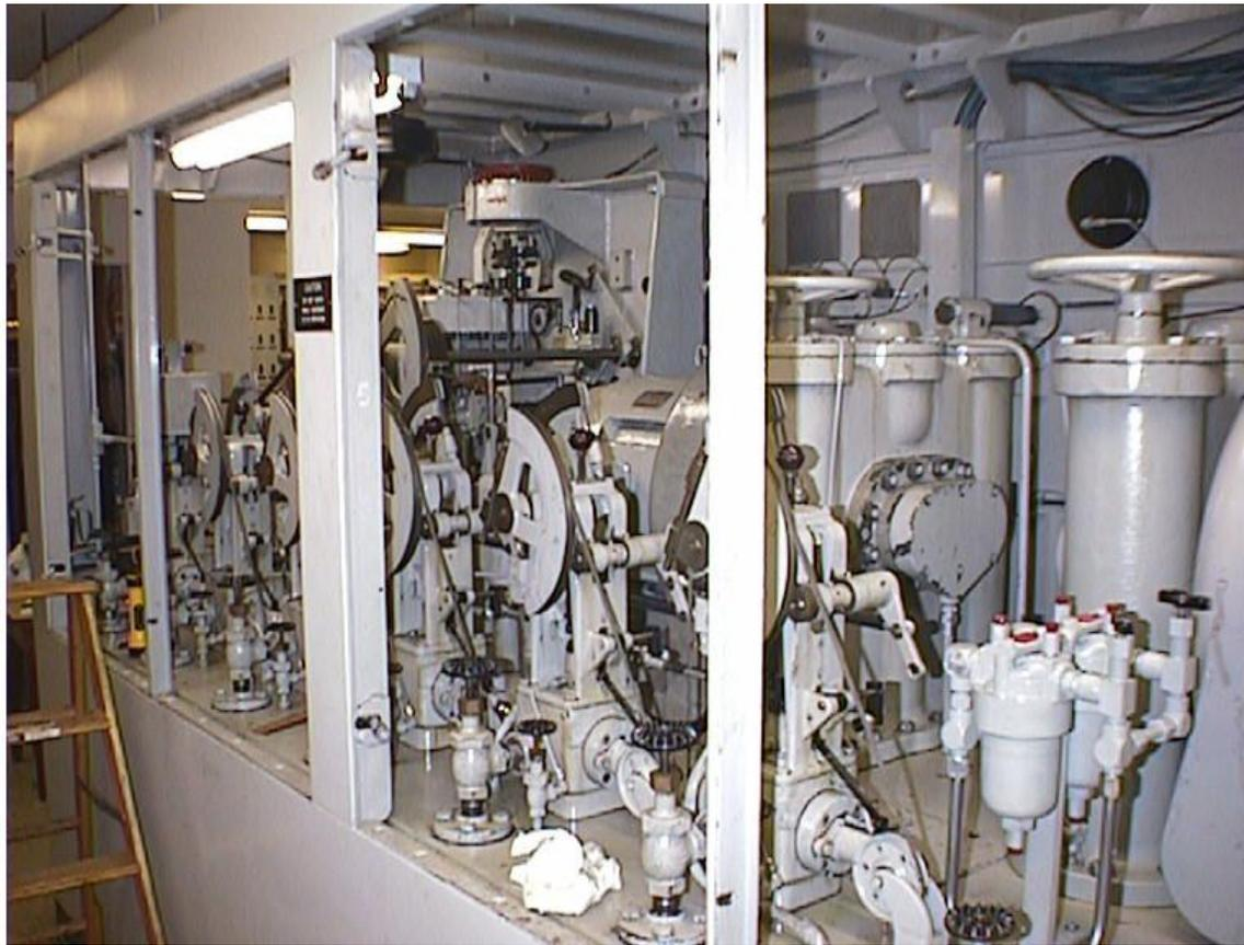
Figure 3 – Woodward Mechanical Governor - 6 Needle Impulse Turbine
