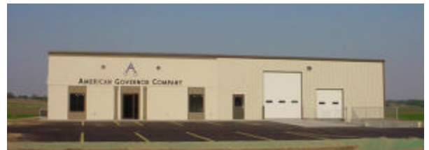
Wisconsin Training and Repair Facility
