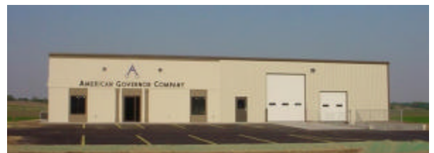
Wisconsin Training and Repair Facility
