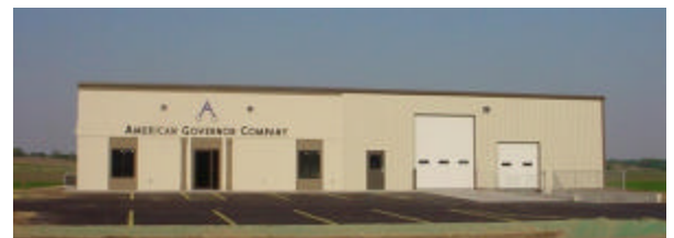
Wisconsin Training and Repair Facility
