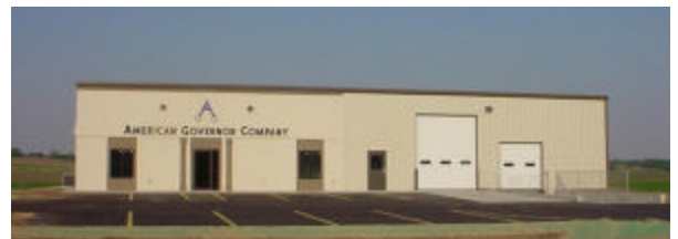
Wisconsin Training and Repair Facility
