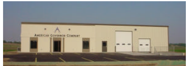
Wisconsin Training and Repair Facility
