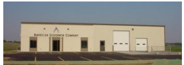
Wisconsin Training and Repair Facility
