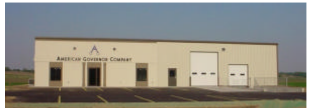
Wisconsin Training and Repair Facility
