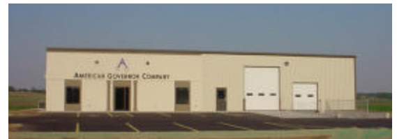
Wisconsin Training and Repair Facility
