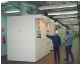
Mechanical Cabinet Actuators
