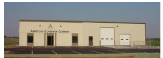
Wisconsin Training and Repair Facility
