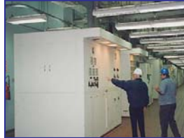
Mechanical Cabinet Actuators
