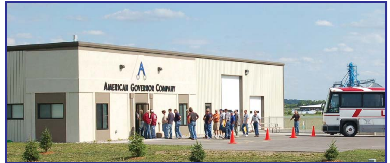
Wisconsin Training and Repair Facility
