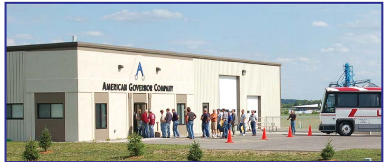
Wisconsin Training and Repair Facility
