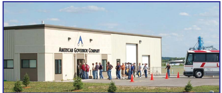
Wisconsin Training and Repair Facility
