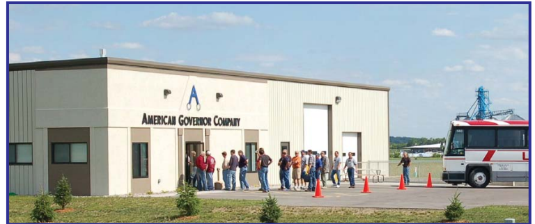
Wisconsin Training and Repair Facility
