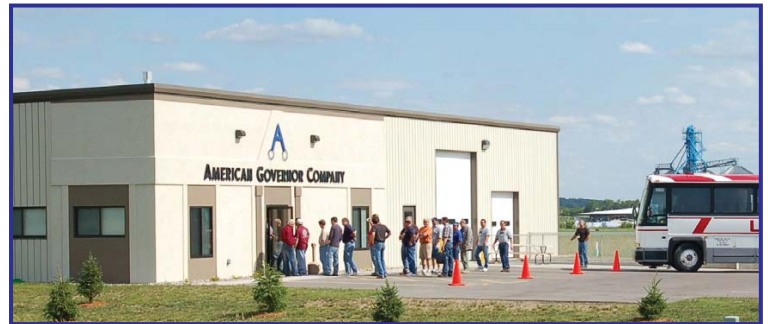
Wisconsin Training and Repair Facility
