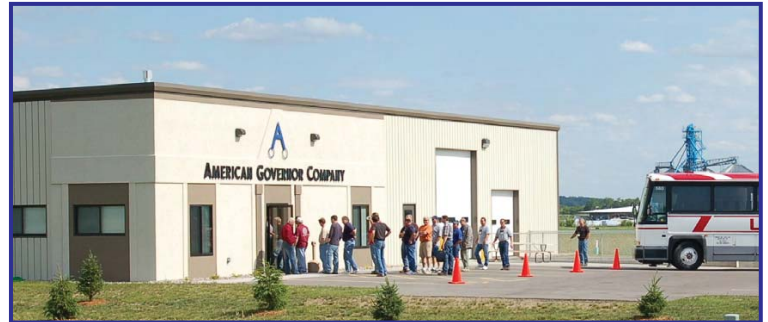
Wisconsin Training and Repair Facility
