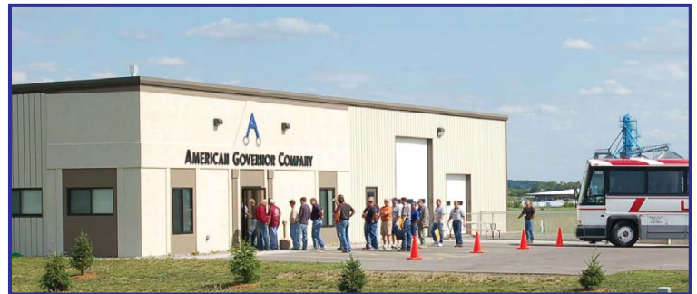
Wisconsin Training and Repair Facility
