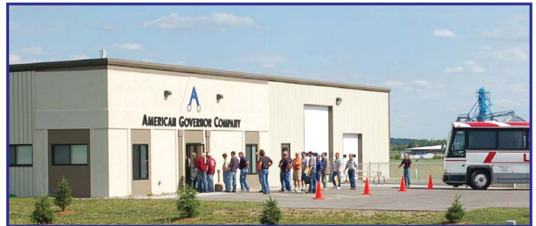
Wisconsin Training and Repair Facility
