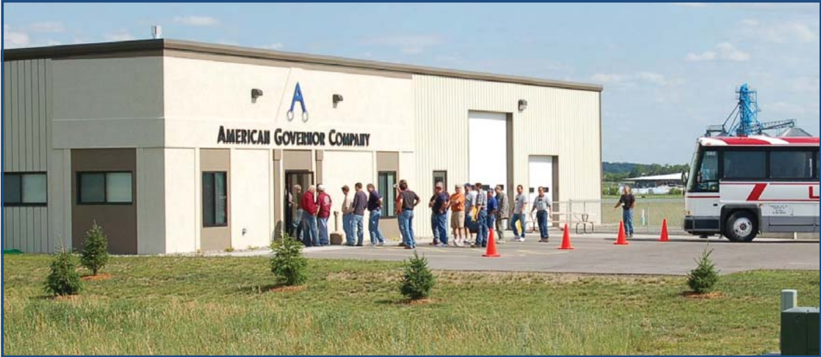
AGC Governor Repair and Training Facility in Amherst, WI
