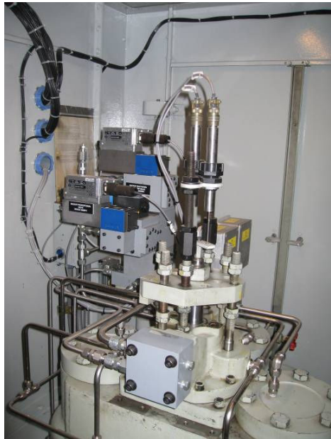
Side and rear views of installed redundant EHI manifold assembly and LVDT feedback devices
