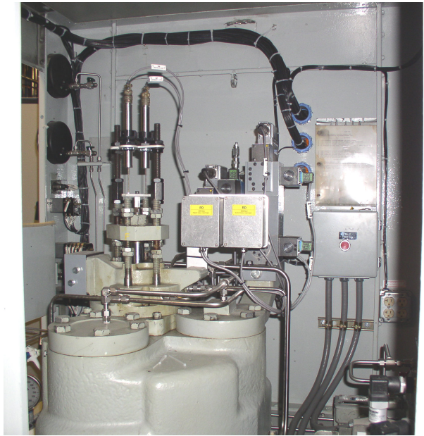
Side and rear views of installed redundant EHI manifold assembly and LVDT feedback devices
