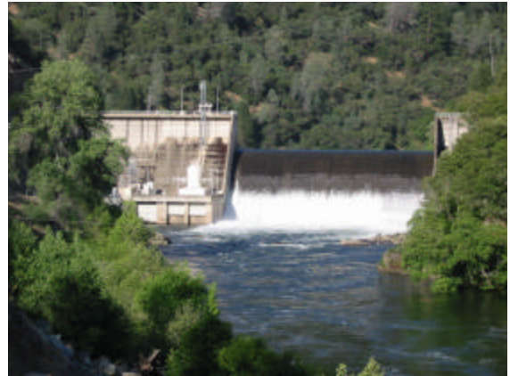
Figure 1 PG&E's Chili Bar plant needed a governor upgrade to meet stringent, new downstream flow requirements.
